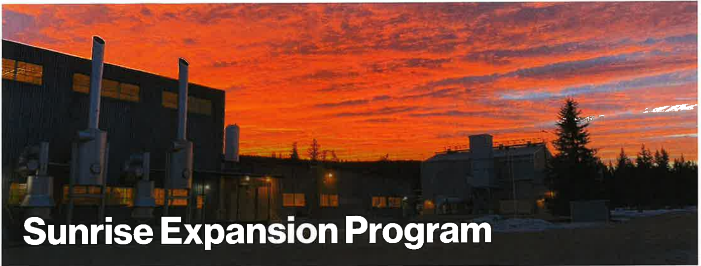
> Image above: existing compressor station 5 – “Australian” – near Quesnel, BC
