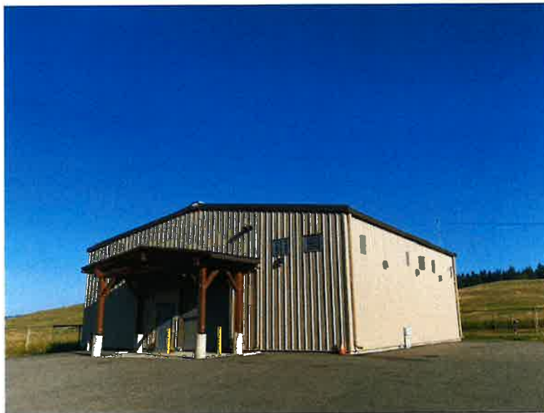
Figure 1: The District of 100 Mile House Water Treatment Plan
